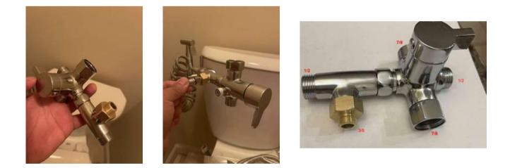
The setup in the above picture was the best I could purchase, but it was too bulky and long to fit in the small space behind the toilet, causing the hose to bend.
